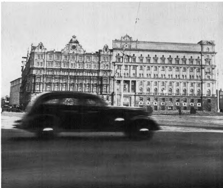
A few months after the Stalin rites, Beria was in Lubyanka prison, a few blocks away. This photo by author is one of few to show famed jail after completion of new building at right
